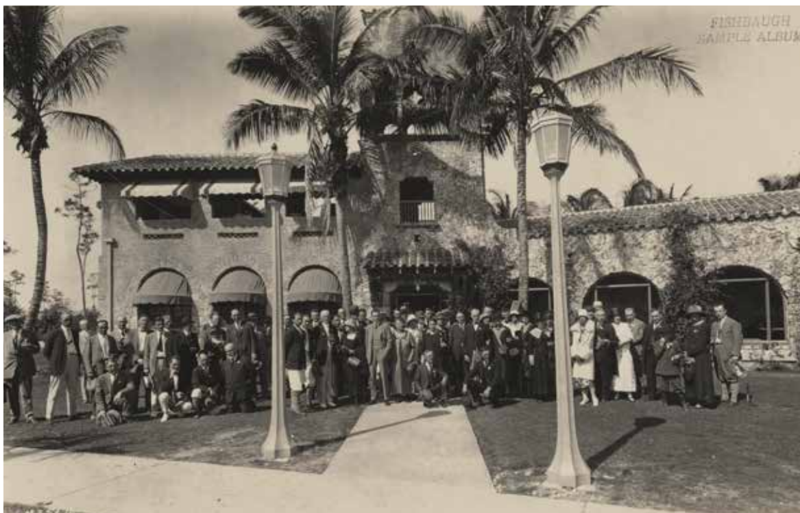
The Coral Gables Country Club in 1925 featured original Arcadian street lights.
